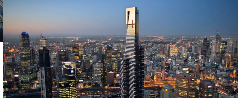
Eureka Tower MELBOURNE - AUSTRALIA
